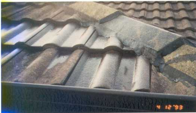
The equivalent product to PROTECTIMBER was applied with a hand held sprayer in 1993.
