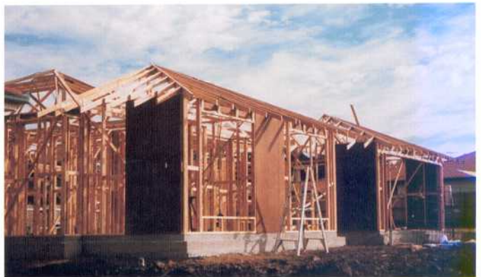
Internally this house can be protected from decay and insect attack by spraying or painting on PROTECTIMBER .
