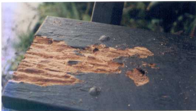
A badly decayed step cleaned ready for PROTECTIMBER application.
