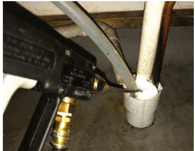
Foam and biological agent being applied to a service drain to sanitise the fly breeding ground
