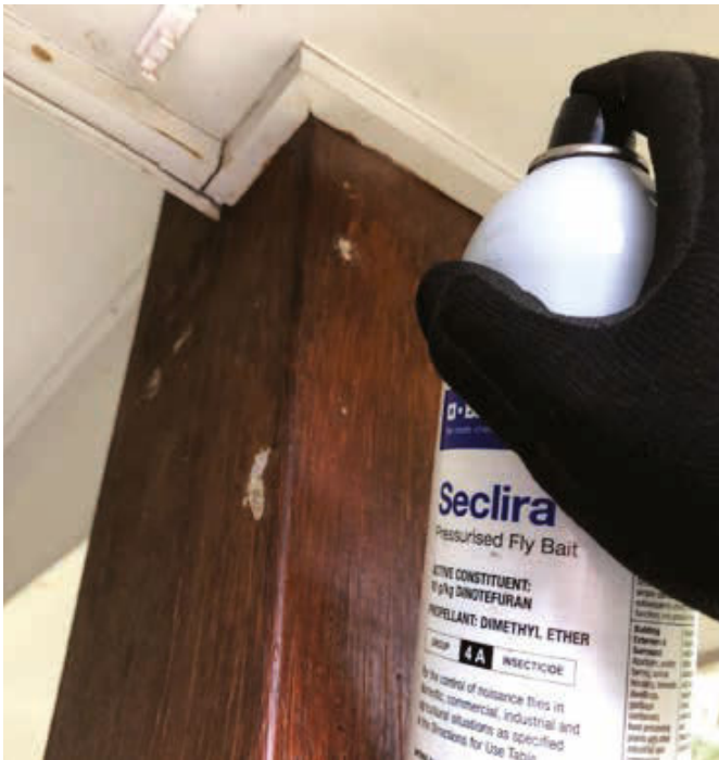
Seclira Pressurised Fly Bait being applied around external pergola supports
